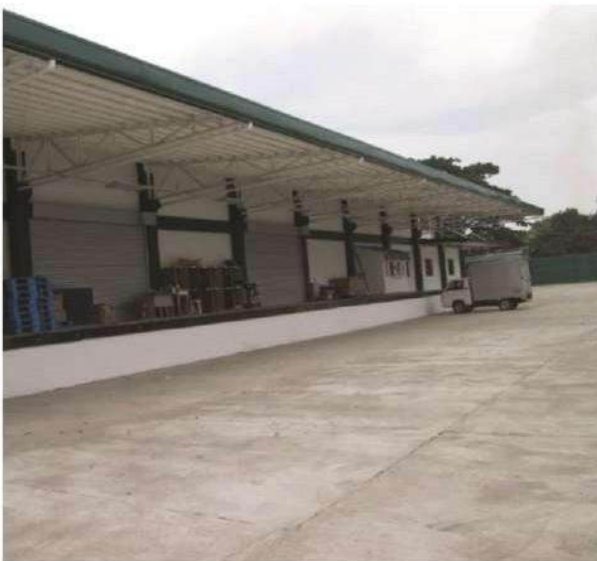
Loading bay for warehouse at Dumaguete sales office depot.
